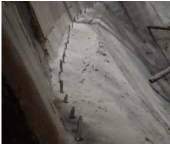
INJECTION GROUTING
