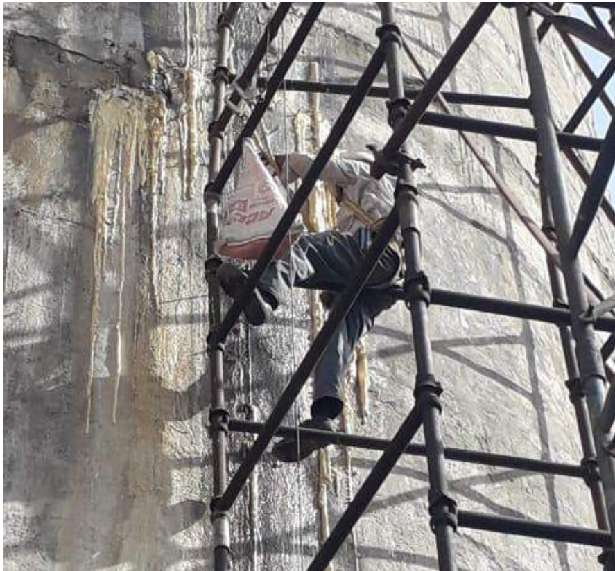
ANAEROBIC TANK PU & CEMENTITIOUS INJECTION GROUTING PANCHAMRUT DAIRY, MIDC TALOJA, MAHARASHTRA
