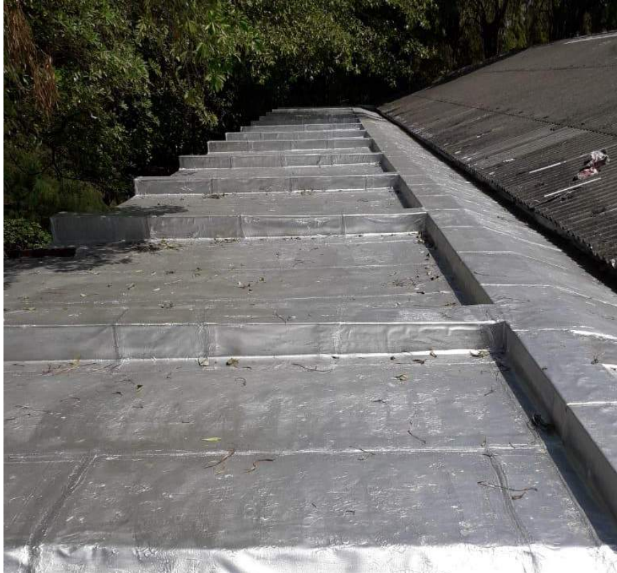
BITUMEN MEMBRANE WATERPROOFING ATUL LTD, GUJARAT
