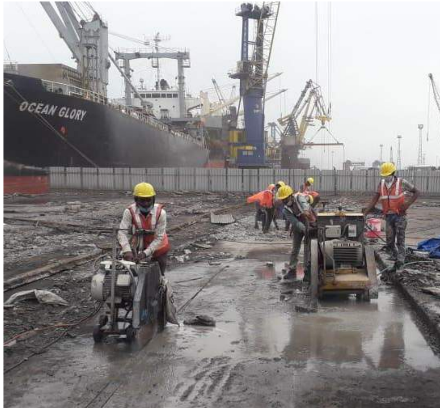
SLAB CUTTING & BREAKING WITH SAW MACHINE DINDAYAL PORT TRUST, KANDLA
